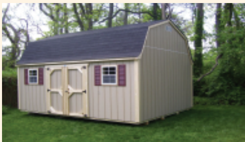
Standard building ready to paint
